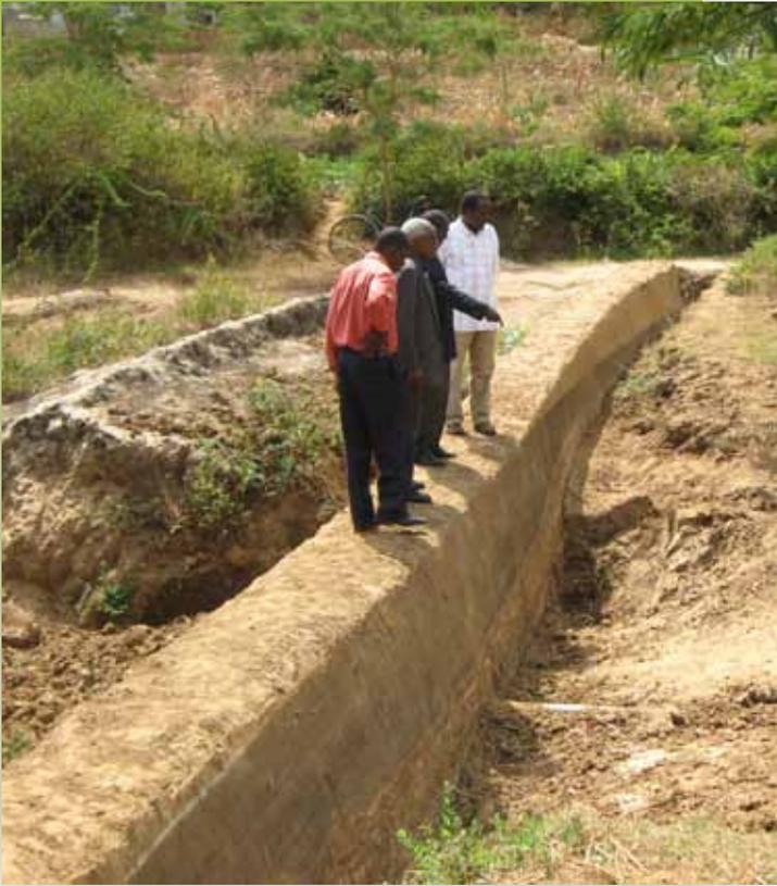
Sand dams constructed in Sakai and other parts of Kenya have proven to be reliable sources of water for people, livestock and plants during the dry season and in times of drought. By slowing the flow of creeks or rivers, these dams trap sand (which prevents evaporation) and cause water to percolate underground, where it remains available for future use.
